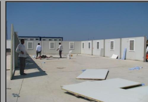
Must be erected on level concrete ground
