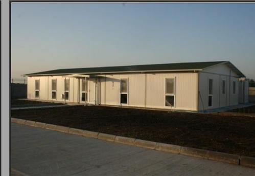
The max. distance between axis can be 4m. which provides flexibility to design buildings according to your
