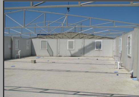
Structure is mainly composed of load bearing columns and trusses
